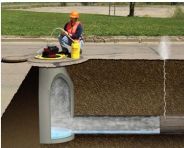
*High-capacity blowers are used to pump smoke into a manhole (left photo). In the right photo, smoke is pushed into the system and emerges from cracks in the service line or missing cleanout cap.*
